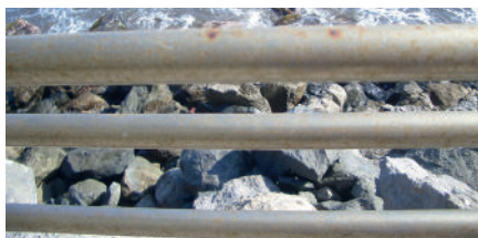
Photo: Maintenance Cleaning of tea-staining of hand railings on the sea side
